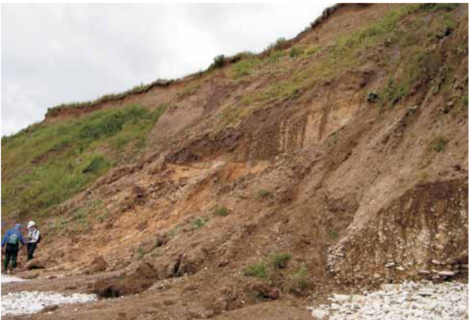
Raised beach deposits and buried cliff at Sewerby. At lower right, interglacial (Ipswichian) shingle beach deposit approx 1m above the current beach. Succeeding unit, bottom left to middle upper right, aeolian sand (Devensian) and finally Skipsea Till with overlying Sewerby Gravels at the top.
