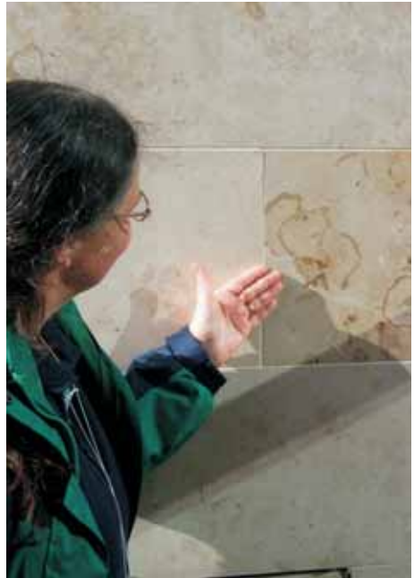
Cardinal House, St Mary's Parsonage. Jurassic Jura Grey Limestone with sections of sponges.
