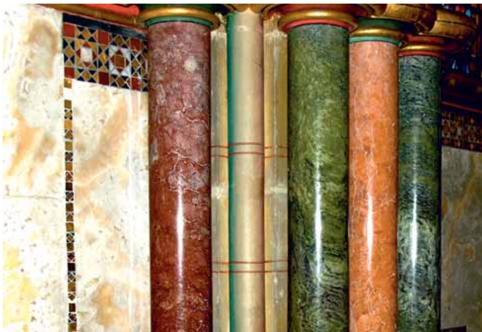
Some of the colourful polished stone with travertine panels and coloured columns.
