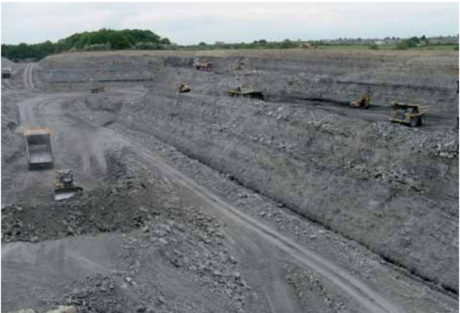
Lodge House Opencast Site showing coal of the Waterloo group of seams being worked; back filling to left.
