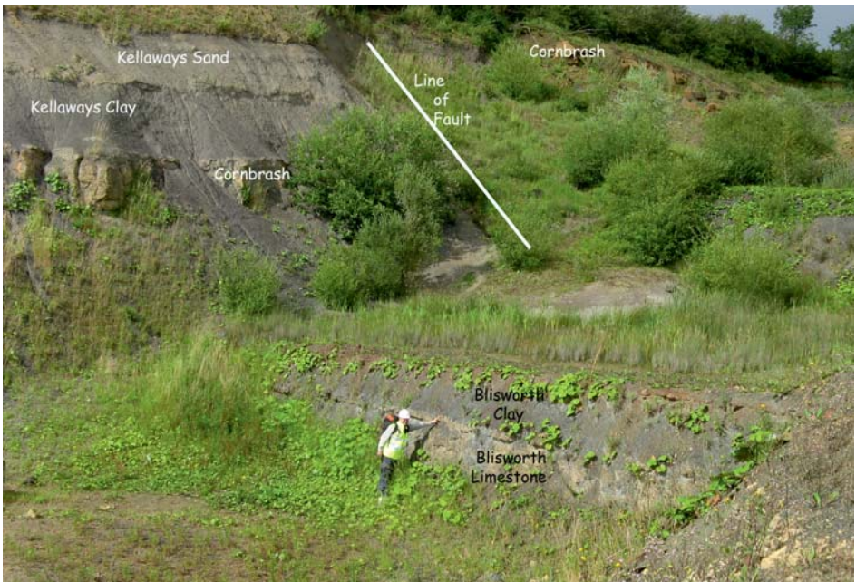
Effects of faulting in Ketton Quarry with the leader pointing to cone-in-cone calcite at the top of the Blisworth Lst.
