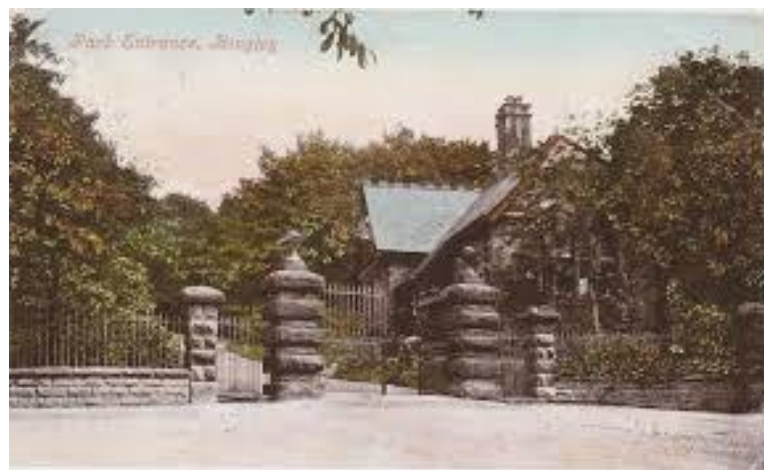
The Park Lodge and Gates
